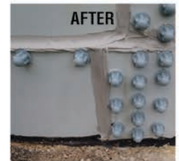
Power Washing, Fillet Replacement and Nut Covers
