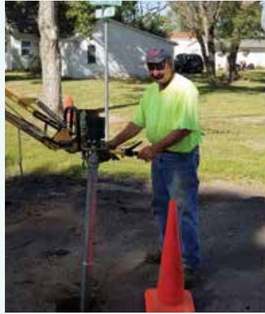
Spinning valves in Pukwana with SDARWS Circuit Rider Jeff Fossum
