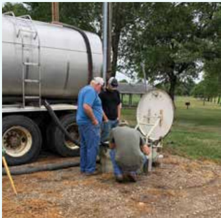
Poly-pigging in Corona, SD with SDARWS Wastewater Tech Danny Ayers
