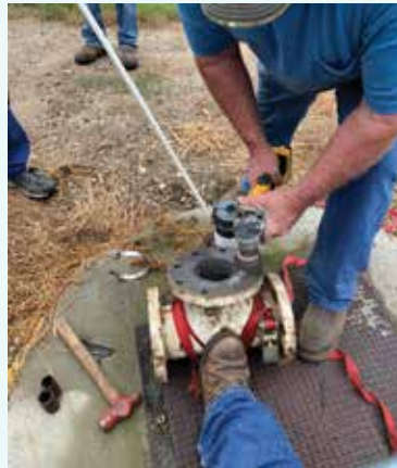
Poly-pigging in Corona, SD with SDARWS Wastewater Tech Danny Ayers
