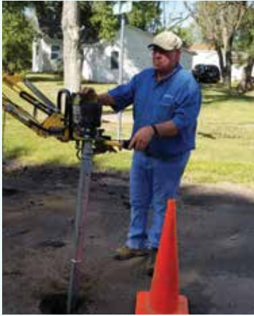
Spinning valves in Pukwana with SDARWS Circuit Rider Jeff Fossum
