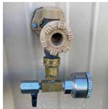
Newer style data logger that SDARWS Uses
