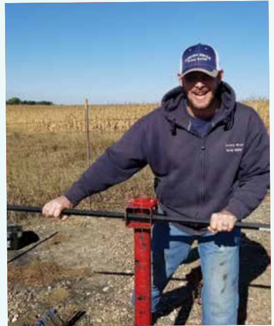
Hydrant repair with a smile at Aurora-Brule RWS
