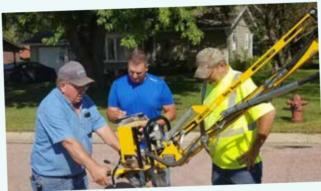
SDARWS Circuit Rider Jeff Fossum in Baltic with City employees, Dan Hotzler and Ken Johnson cleaning valve boxes and exercising valves.
