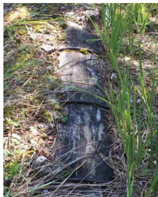
This exposed wooden pipe is thought to be 120 years old!
