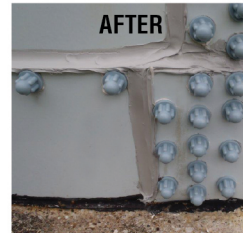
Power Washing, Fillet Replacement and Nut Covers
