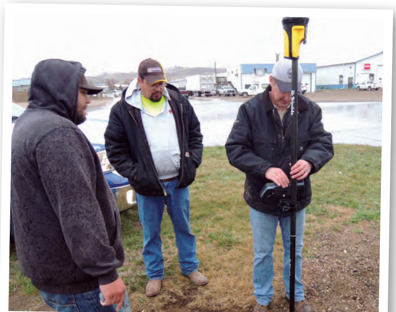
Mike Moeller collecting GPS coordinates of a curb stop.
