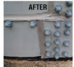
Power Washing, Fillet Replacement and Nut Covers
