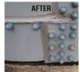
Power Washing, Fillet Replacement and Nut Covers
