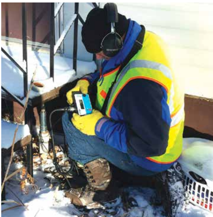
Circuit Rider Nick Jackson using locator to find curb stops under the snow
