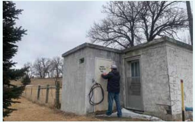
Source Water Protection Specialist Kevin Christensen posting tampering signs on Flandreau's wellhouse as a part of their source waer protection plan.
