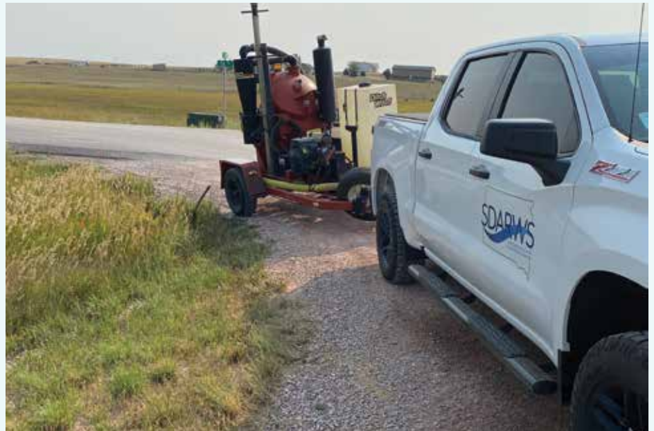
Valve Riser cleaning at Sunset Ranch Estates with the hydro vac.
