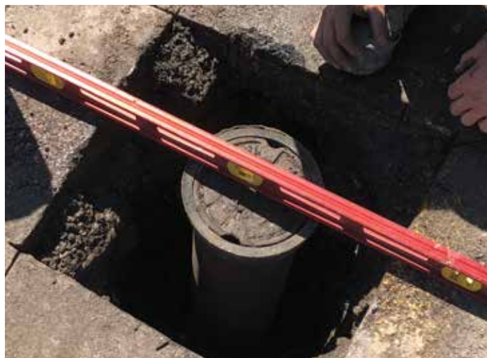
Repairing the valve riser
