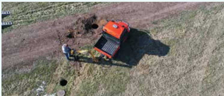
Bill Thorson takes selfies to new heights! Here he is using the valve exerciser to assist with an emergency valve repair at the lagoons in Viborg.
