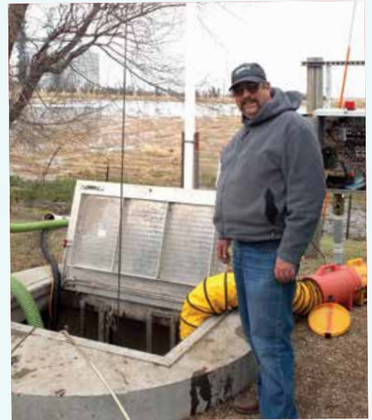
SDARWS Wastewater Tech Danny Ayers assists with poly pigging in Seneca.
