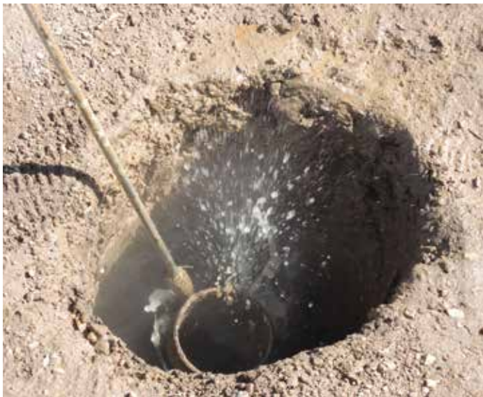
Power washing the soil into a slurry around a valve riser.
