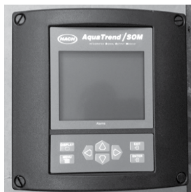
Hach AquqTrend/SOM Integrated Signal Output Module P/N 51350-60
