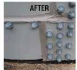
Power Washing, Fillet Replacement and Nut Covers
