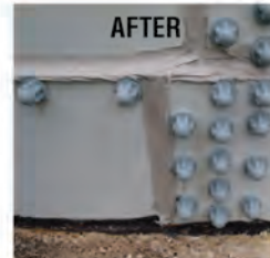
Power Washing, Fillet Replacement and Nut Covers
