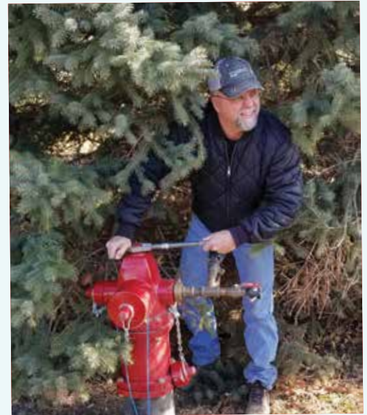
SDARWS Circuit Rider Greg Gross doing leak detection in Faulkton.
