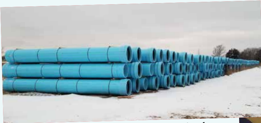
20,000 feet or 3.79 miles of 24-inch pipe ready for relocation of a waterline by the Randall Community Water District.
