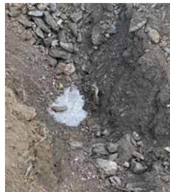
Water surfacing in the bottom of the trench.
