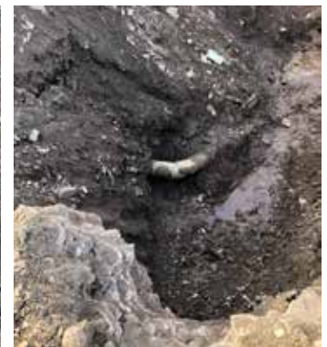
Repaired cast iron line.
