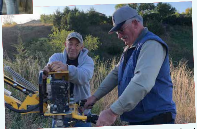
Nick Jackson helping exercise 30-year-old water main valves in Chamberlain with Public Works Supervisor Brad Mohror.
