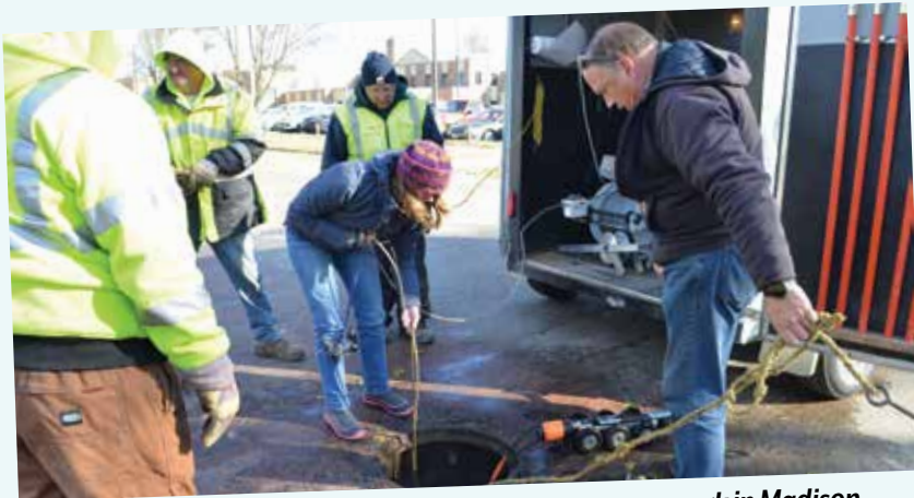
Abbey Larson and Bill Thorson doing sewer camera work in Madison.
