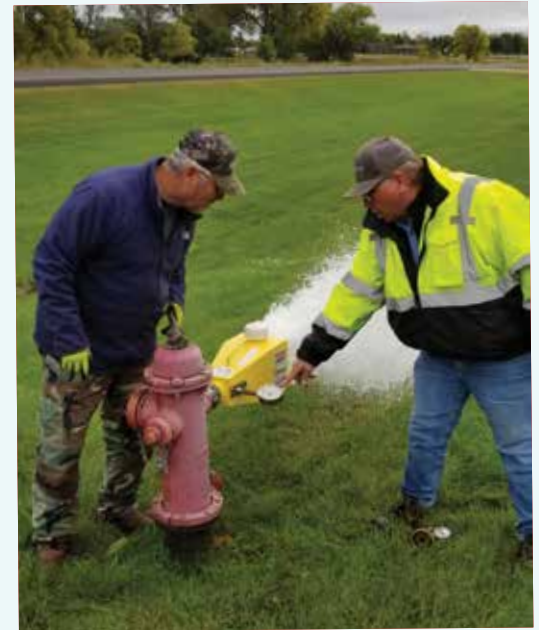
Jeff Fossum assisting with hydrant flushing in Howard.
