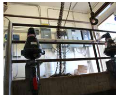
View of new lift station in Winner, SD. Improvements include new controls, air relief valves, and check valves.
