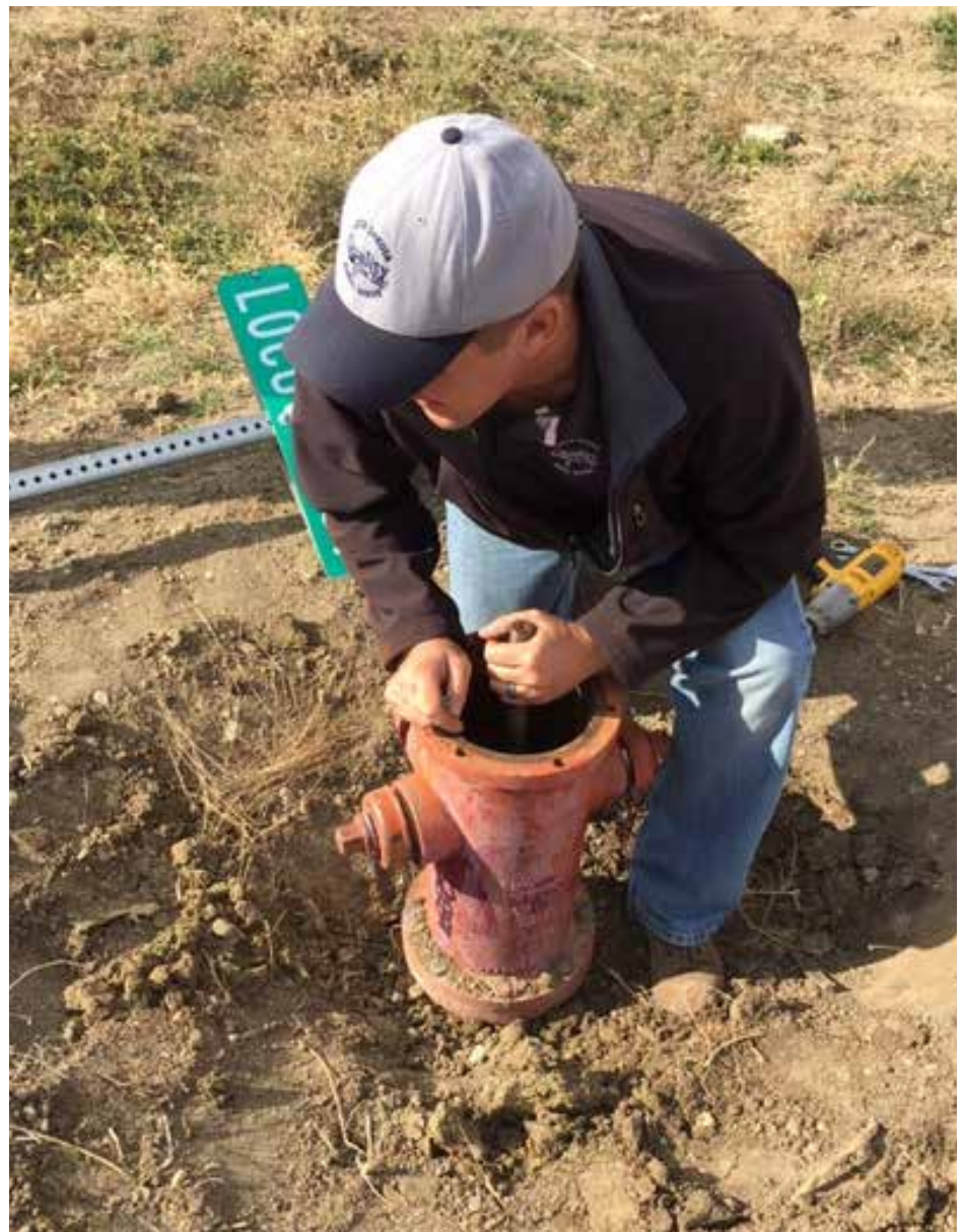
SDARWS Circuit Rider Mike Moeller working on dismantling a hydrant.
