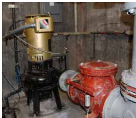
View of new lift station in Winner, SD. Improvements include new controls, air relief valves, and check valves.
