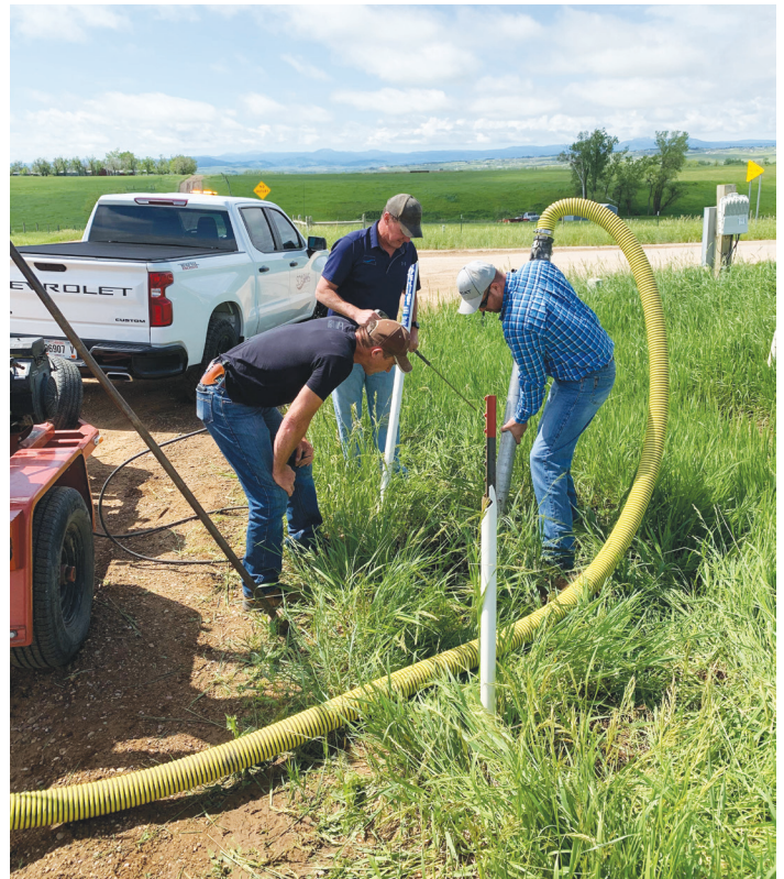
Excavating a valve riser with the hydro-vac.
