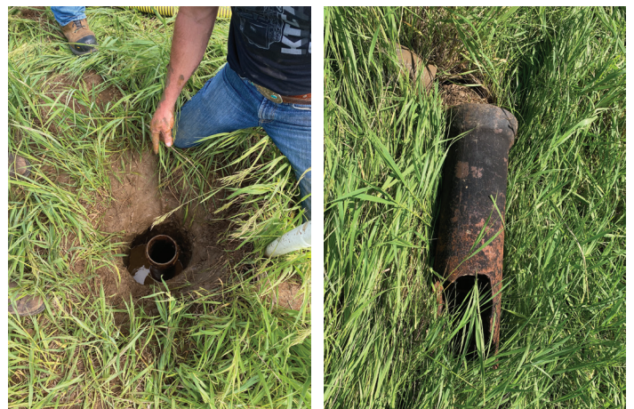
Top section of valve riser removed.
