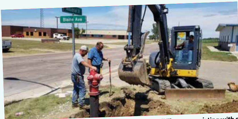
SDARWS Training/Technical Assistance Specialist Bill Thorson assisting with a fire hydrant replacement in Viborg.
