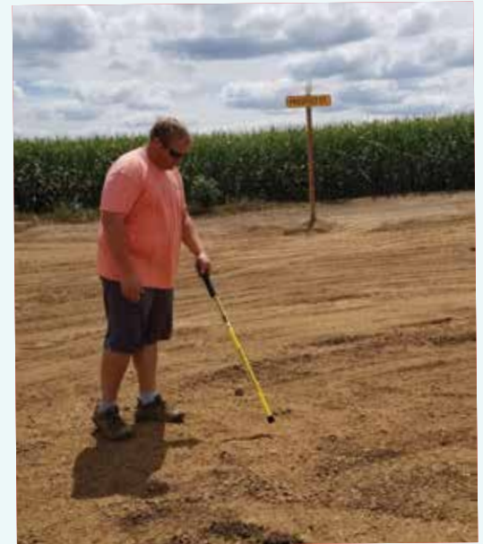
SDARWS Circuit Rider Jeff Fossum assisting Colman operator Grant Groos GPS valves.
