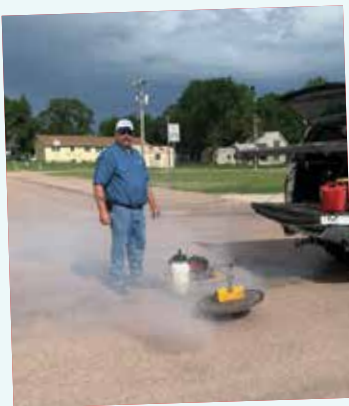
Wastewater Tech Danny Ayers smoke testing in Mt. Vernon.
