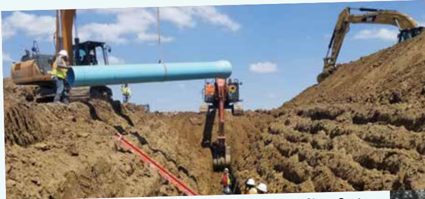
Lewis & Clark Regional Water pipeline construction near Sioux Center.
