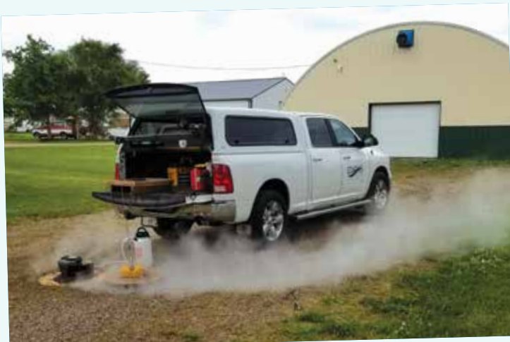
SDARWS Wastewater Tech Bill Thorson smoke testing in Menno.
