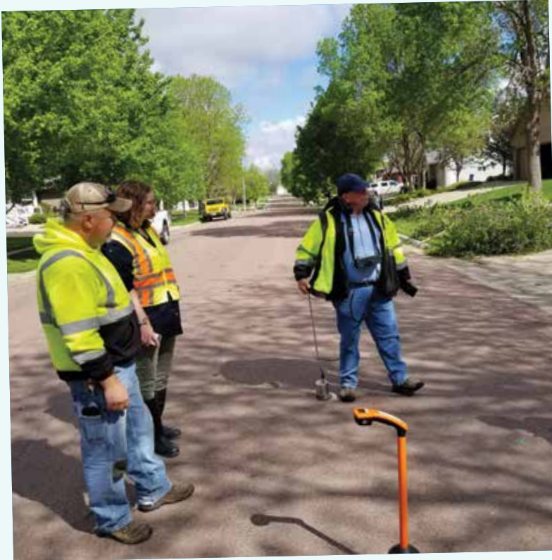
Circuit Rider Jeff Fossum out finding leaks in Brandon.
