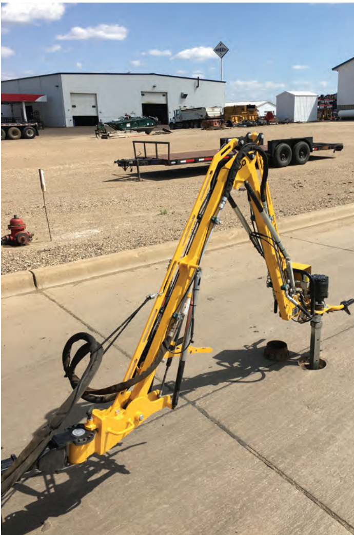
Exercising valves on hydrant legs.
