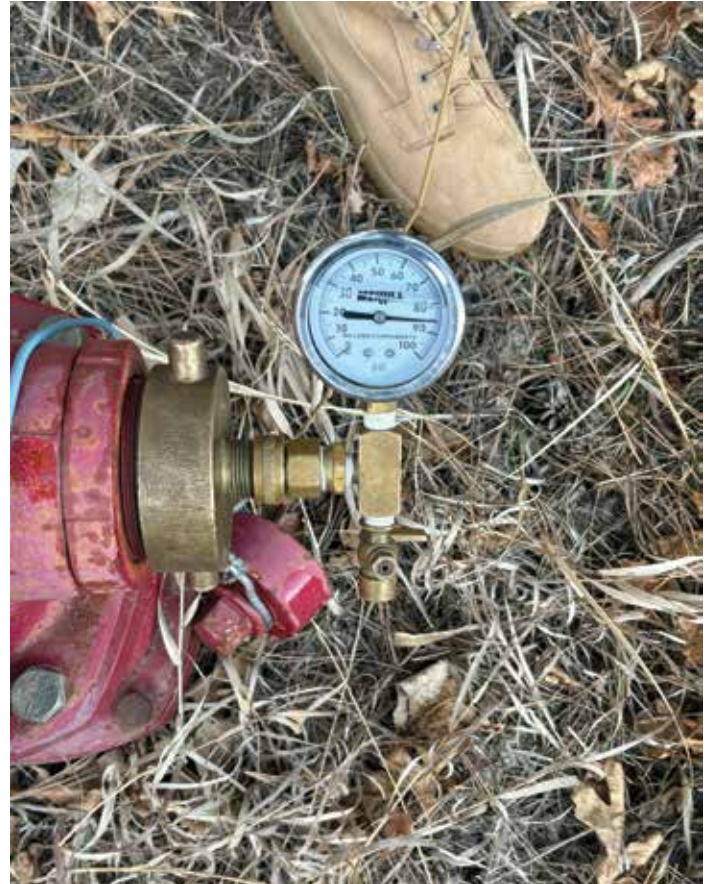
Static pressure being recorded in system
