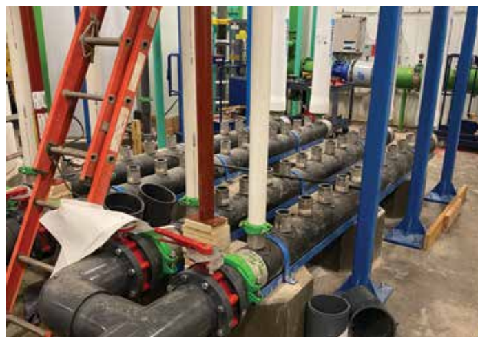
Rebuilding the headers to accommodate the new filter cartridges
