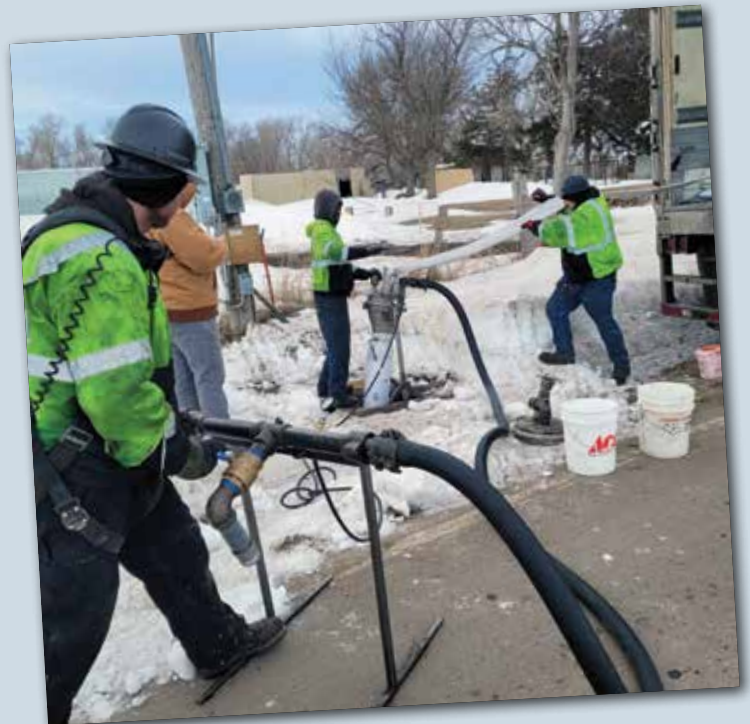
Pipe relining project in Delmont.
