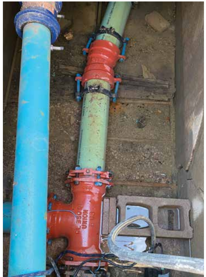
Vault with water below tank
