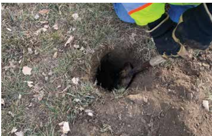
This curb stop was found 18+ inches below the surface.
