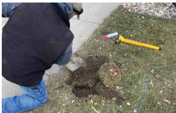
Uncovering a curb stop after tracing it.
