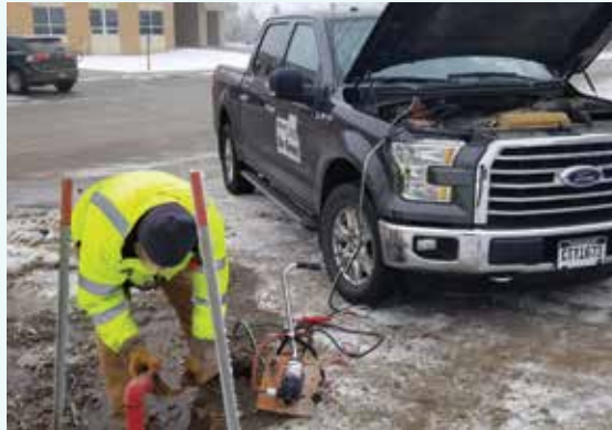
SDARWS Circuit Rider Jeff Fossum was in DeSmet assisting Operator Charlie Stoddard with flushing a dead-end water line in winter.
