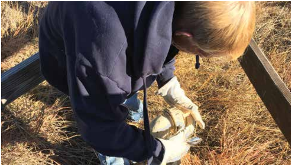
Checking for chlorine residual along the main
