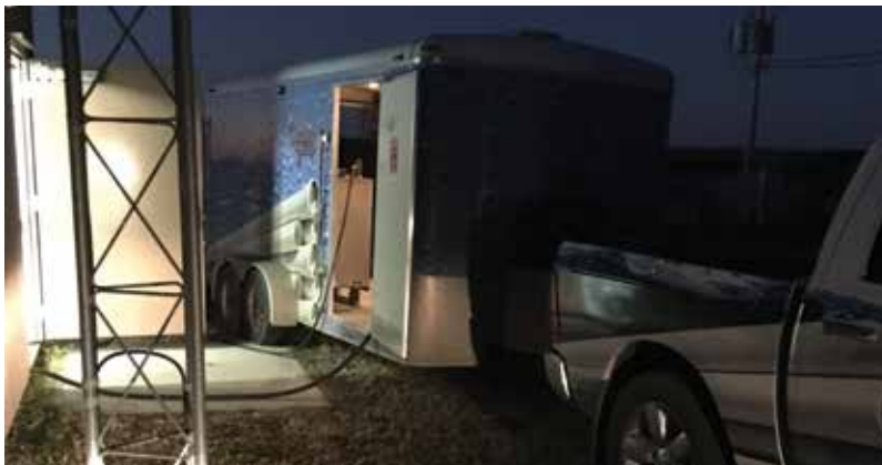
Leak detection trailer hooked up to pump station and hose running to the chlorine injection point.
