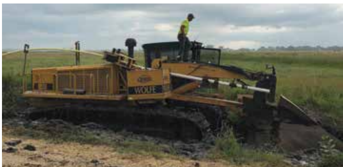
Installing over 200 miles of project mainline pipe using plowing technology.
