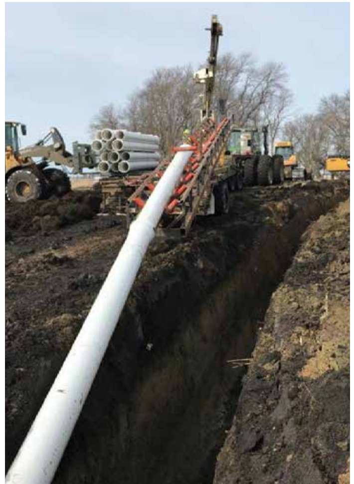
12-inch diameter pipeline installation.
