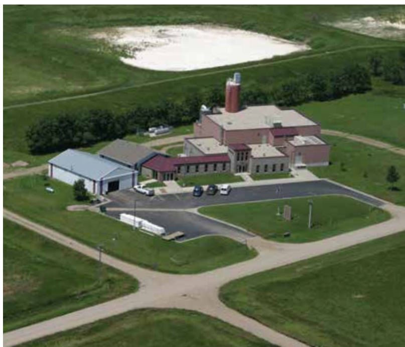
Aerial view of the Big Sioux Community Water System plant near Egan, SD.
