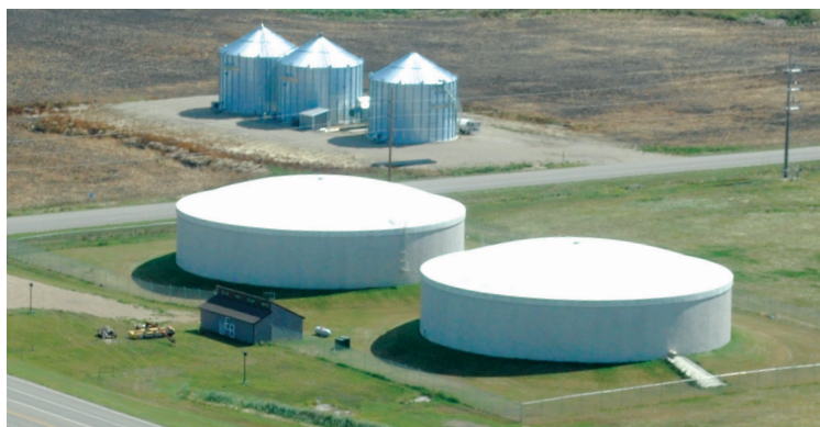
Page 6, from L to R: Elevated Riveted Tank, Pedestal Spheroid Tank, Composite Tank, Elevated Tank, Steel Ground Storage Tank. Below: Ground Storage Tank. Right: Pedestal Spheroid Tank.
