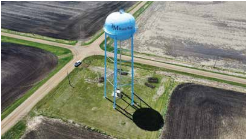
Aerial view of TM Rural Water tower
